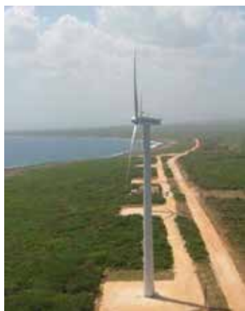
Wind park at Gibara
